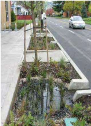
Tree Basin - an example of LID that allows stormwater runoff to infiltrate into the soil, thereby reducing runoff volume and peak flows.
